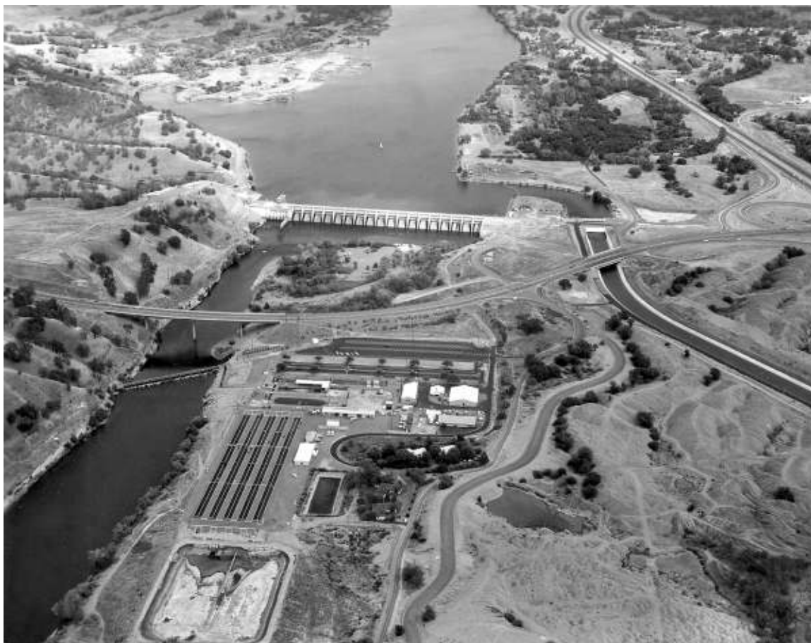
Figure 1-13 Oblique aerial photo of Nimbus Dam and Fish Hatchery (photo: J.C. Dahilig, Bureau of Reclamation, 10/4/1976)
