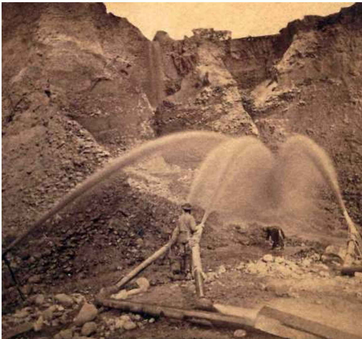
Figure 1-11 Hydraulic mining in the Sierra Nevada (Photo: Central Pacific Railroad Photographic History Museum)
